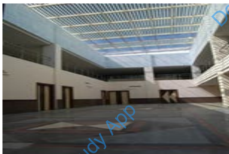
BIPV in Roof
