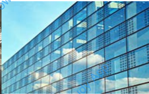
BIPV in Facade
