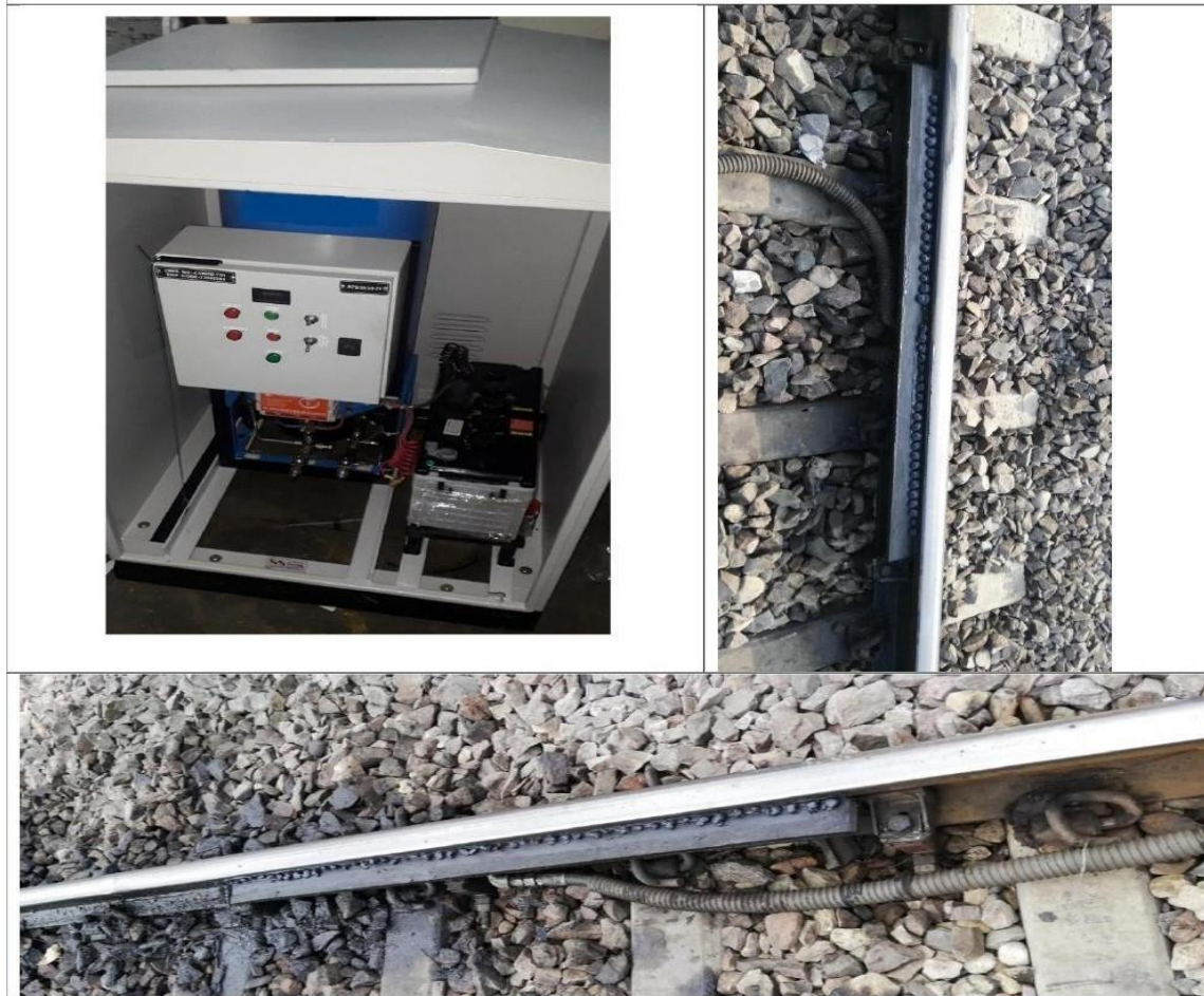
Track Based Lubricator (Electronic Type )
