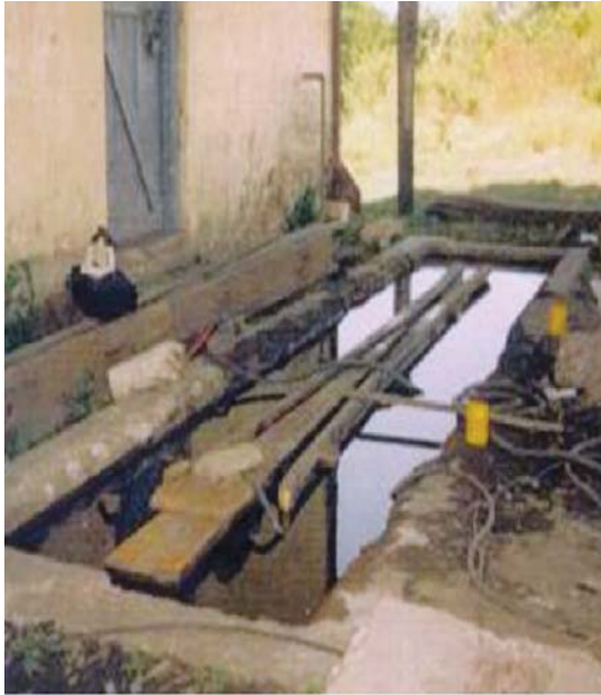
Fig. 6.2 Reconditioning of CMS crossing
