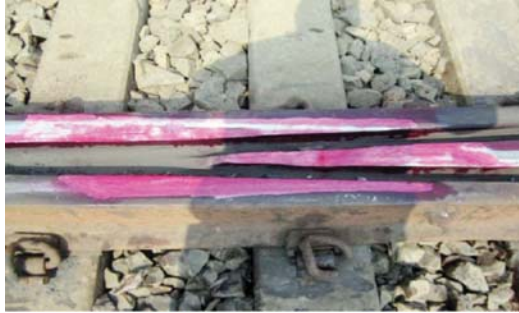
Fig. 6.4 Dye penetration test
