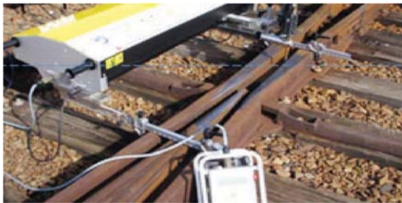
Fig. 6.3 Translamic Robotic welding
